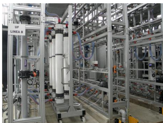
Figure 4. Outside-in pressurized ultrafiltration membranes installed in a rack and its module
