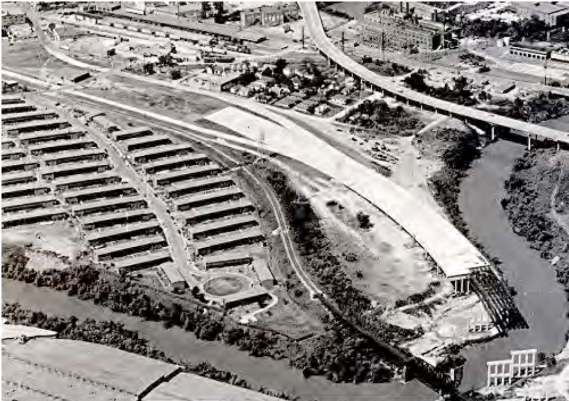
Schrimpf's Field, circa 1955, with the Clayton Homes and US 59 construction. Photo courtesy of TxDOT.
