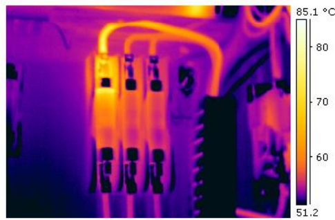
Figure 5.2.: Electrical fault
