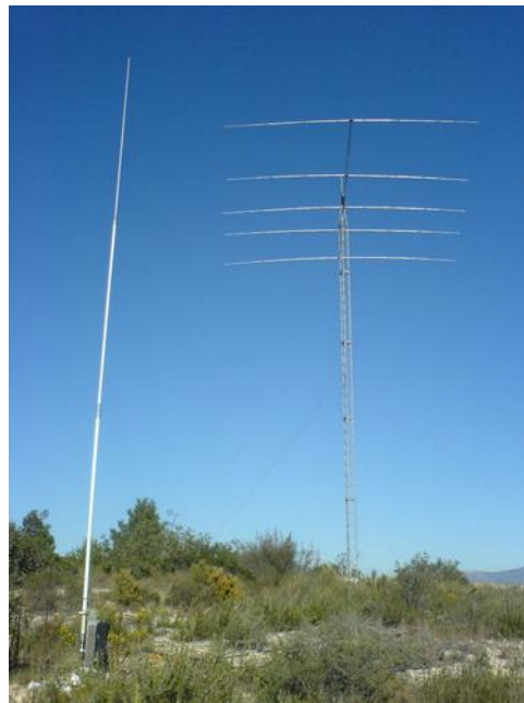
FIGURE 3.5: The installations of yagi and monopole antennas at OE during 2009/2010.
