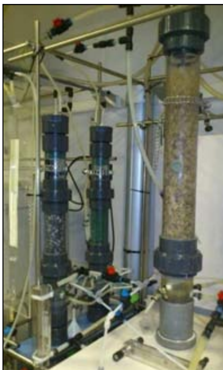
Figure 4.3. Image of the desulfurizing BTF system
