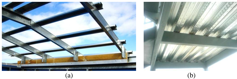
Fig. 1.6 (a) Hat sections about to bear roof in a warehouse; (b) Structural roof deck
