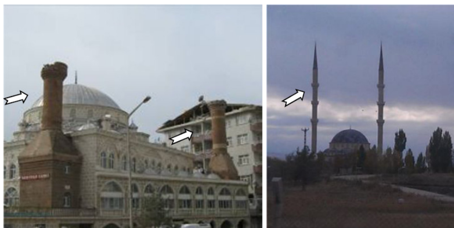
e) Collapse of historic minarets in Van (Turkey) at the weaker section at balconies (Ozturk, 2013)
