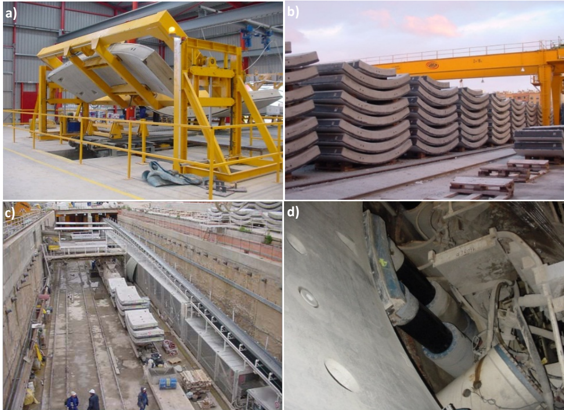
Figure 2.1 Temporary load stages of a segment: a) demoulding b) stocking, c) transport and d) thrust of jack
