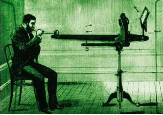
Fig. 6: Photophone Transmitter and receiver, after [6]
