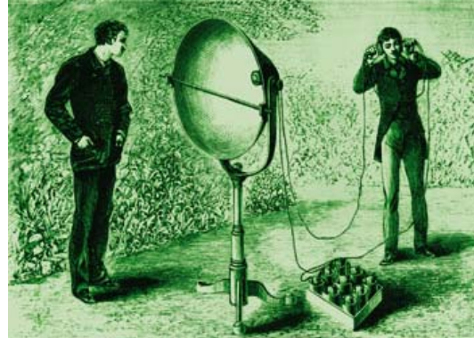
Fig. 6: Photophone Transmitter and receiver, after [6]
