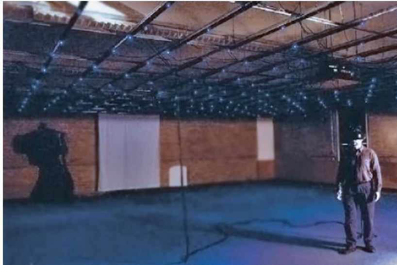
Figure 3-2 An array of Intersense IS-900 at Brown University. Figure adapted from [Tarr and Warren 2002].
