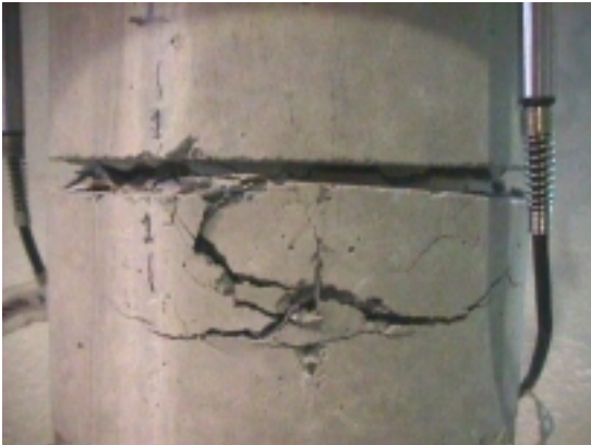
Figure 2.7. Crack deviation outside the notch
