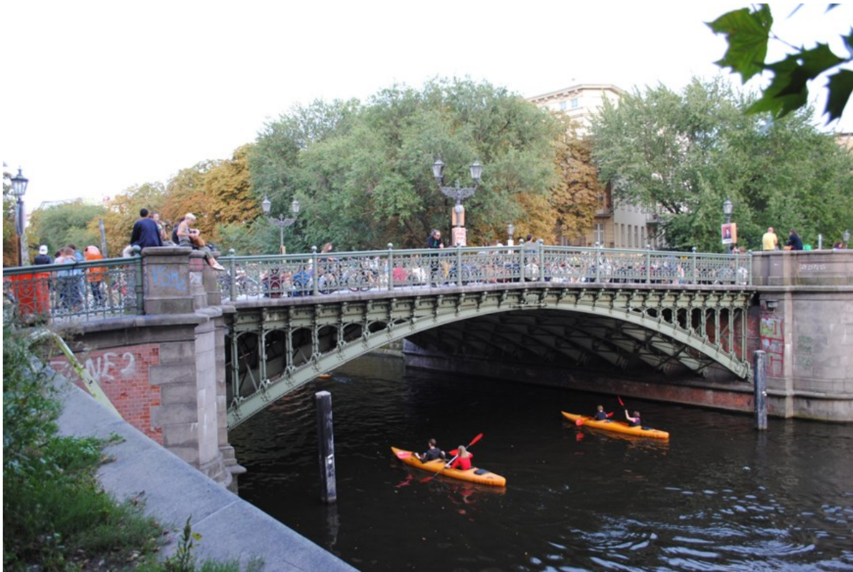
Figure 3: View of the bridge from the north-west shore (Author, 25.08.2017, 19:47h)
