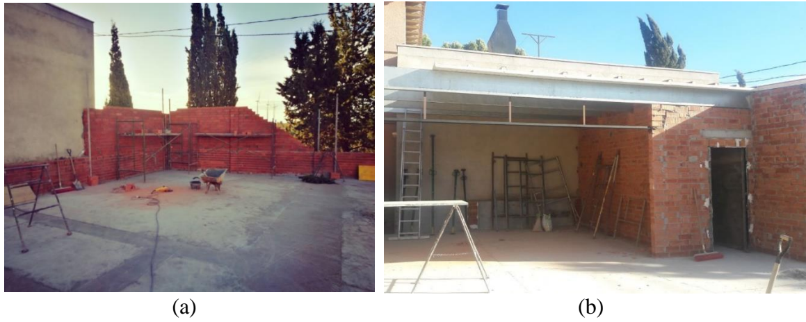
Figure 8. Building process. (a) engine room; (b) control room.
