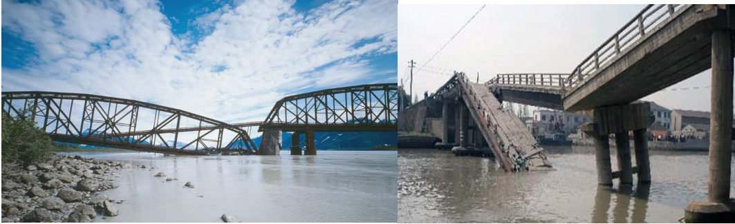
Figure 1-1. Some examples of bridge collapse
