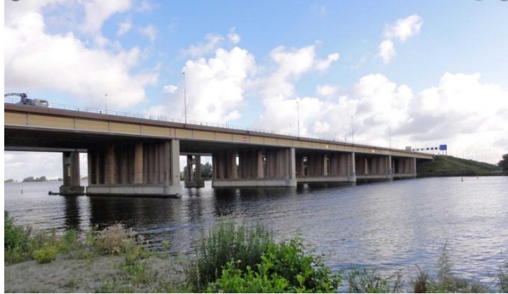
Figure 4-8. Overview of Hollandse Brug
