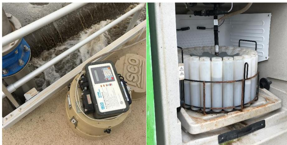
Figure 6 Wastewater treatment plant autosamplers
