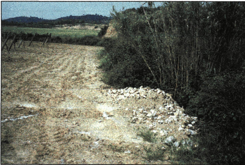
Figure 4.26. Stack of stones in the boundary between a gully and a parcel in order to avoid the retreat of the gully sidewall.
