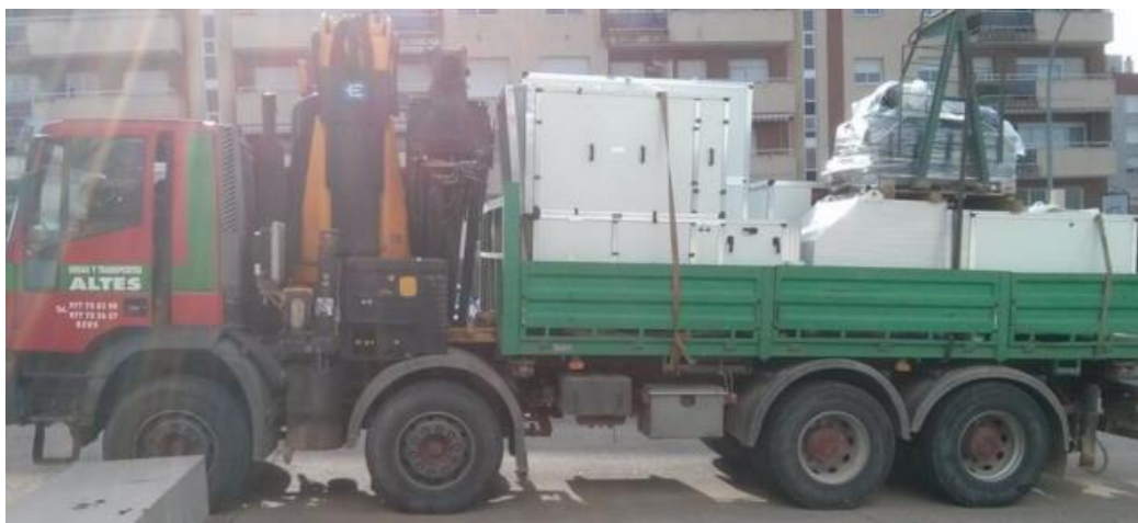
Figure 6.14. Delivery of the air handling unit and the electrical panel.
