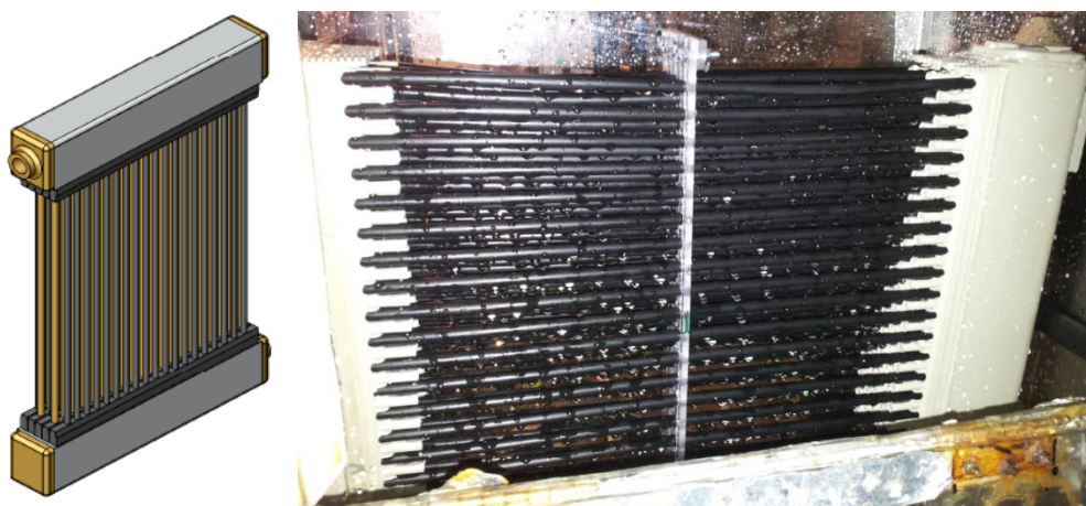
Figure 4.2. Falling-film air-solution contactor.
