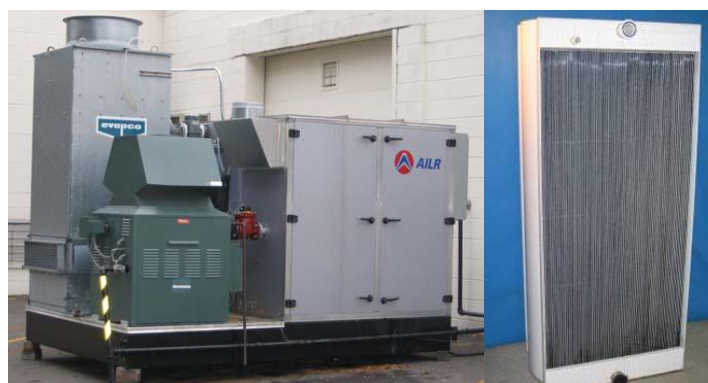
Figure 2.33. Prototype of a 10,200 m 3 /h rooftop liquid-desiccant air conditioner and liquid-desiccant conditioner. AIL Research, Inc. [68].
