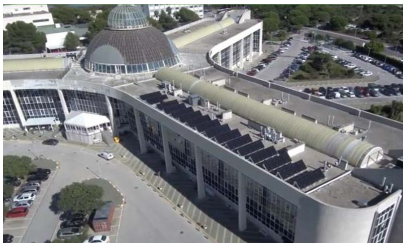
Figure 2-13. Uncovered PV/T collectors installed in Spain (Setolazar Spanish manufacture) [106].
