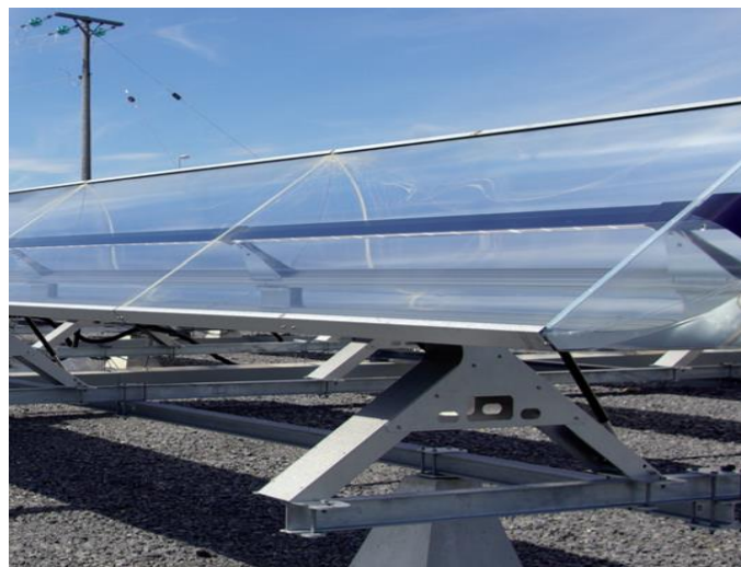
Figure 2-15. Low concentrating Absolicon X10 PVT to generate heat for the district heating network and electricity for the electric power grid installed in Sweden [108].
