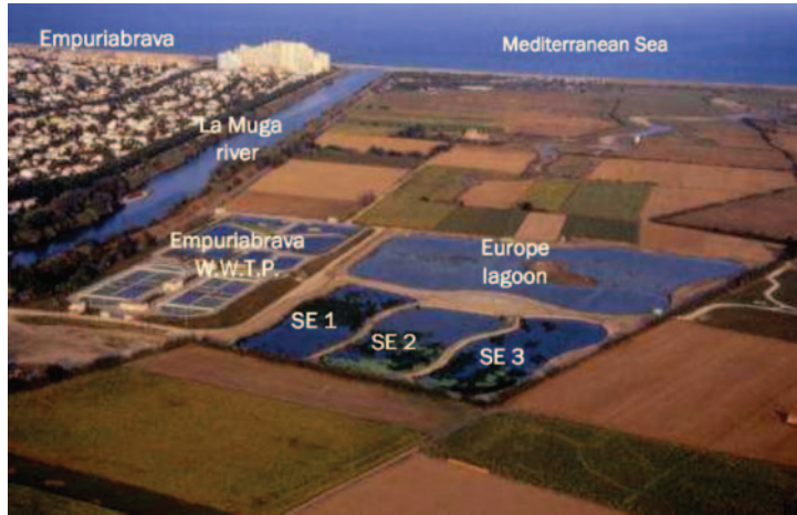
Figure 2.5 Panoramic view of Empuriabrava wastewater treatment plant and the associated tertiary treatment wetlands.
