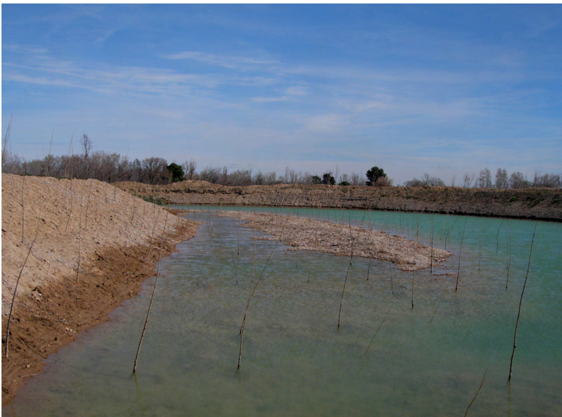
Photo 10. COL creation in abandoned areas of the floodplain to mitigate wetland loss.
