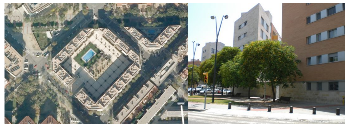
Figure IV.29: residential project in the Olympic Village, Avinguda del Bogatell, Poblenou, Barcelona (Spain): planned long depth sequences
