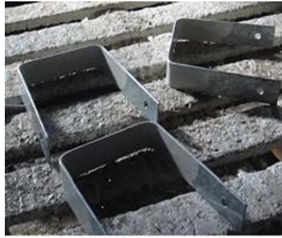
Fig. 1. U-shape anchor system.
