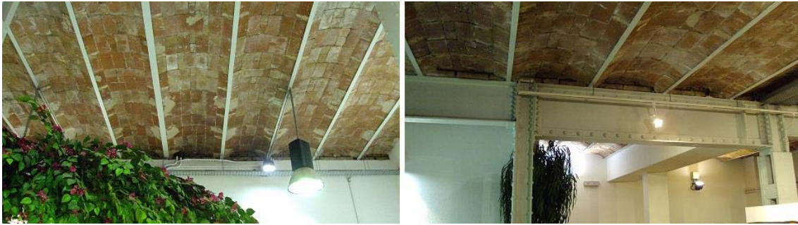
Fig. 1. Typical bottom view of the slabs studied.
