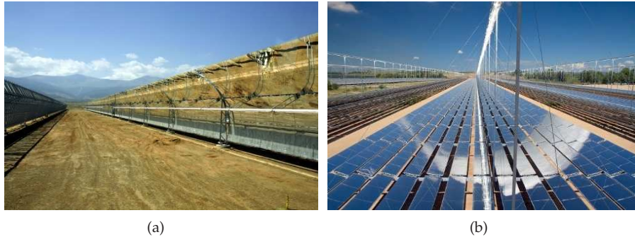
Figure 1.1: Line concentrating systems: (a) Parabolic trough collector: 50 MW power plant Andasol 1 in Granada, Spain [2] , (b) Linear Fresnel collector: 9 MW solar field at Liddell Power station, Australia [3]
