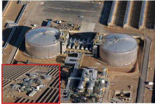
Figure 1.6: The two-tank storage system in the Andasol-1 plant [19]
