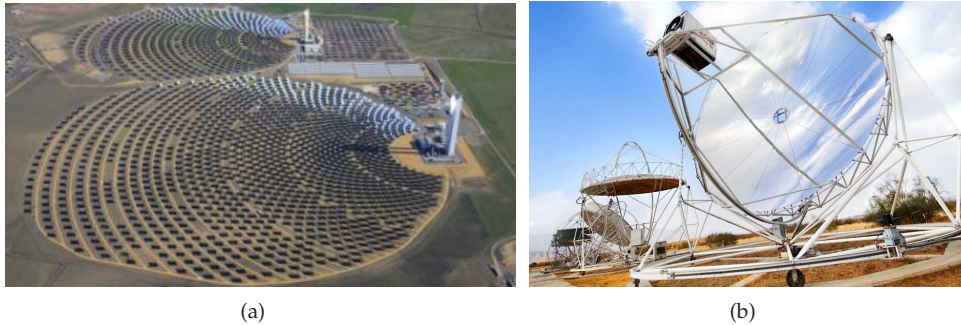
Figure 1.2: Point concentrating systems: (a) Central receiver system: Solar tower plants: PS10 (11MW) and PS20(20MW) in Seville, Spain [7], (b) Dish Stirling prototype plants at Plataforma Solar de Almera, Spain [8]
