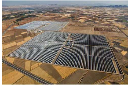
Figure 1.3: Parabolic trough power plants Andasol 1 (in front) and Andasol 2 (rear) in Spain with a capacity of 50 MW each and a storage size of 7.5 hours [2]
