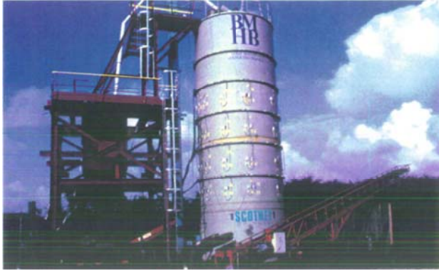
Figure 1-4. Facilities built for the experimental discharge of a full scale silo [89].
