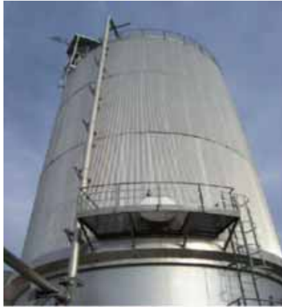
Figure 1.14 Anaerobic digester (DRANCO technology) Source: Juniper Consultancy Service (2005)
