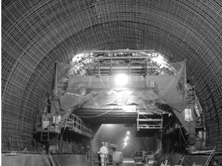
Figure 3.28. Steel reinforcement in vault and abutments of Lilla tunnel
