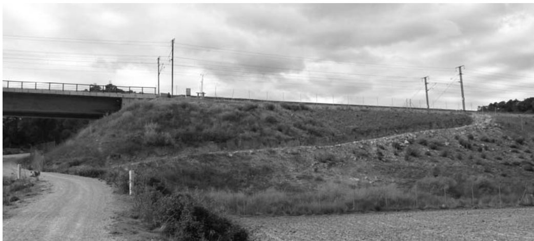
Figure 8.2. Pallaresos embankment, Lleida side. The excavated pathway on the embankment side was made to allow access of drilling machines for the installation of measuring instruments
