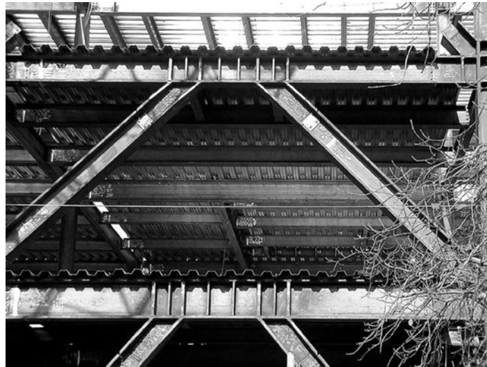
Figure 2-46. Links of an eccentric braced frame
