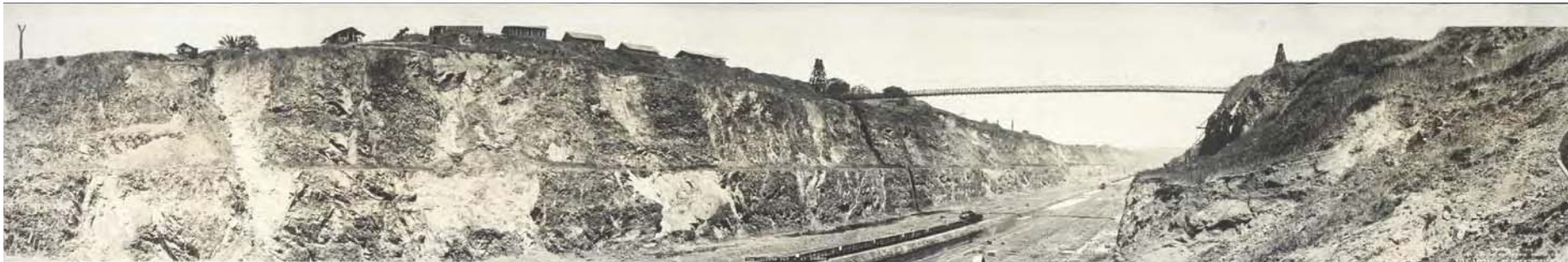
Figura 2.34. Gordon Panoramic Photo Company. Panama Canal. Culebra Cut at Empire , c.1913. © Washington: Library of Congress Prints and Photographs Division.
