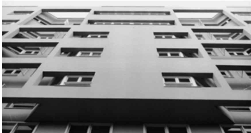
[[Il.d.7] Façana principal
