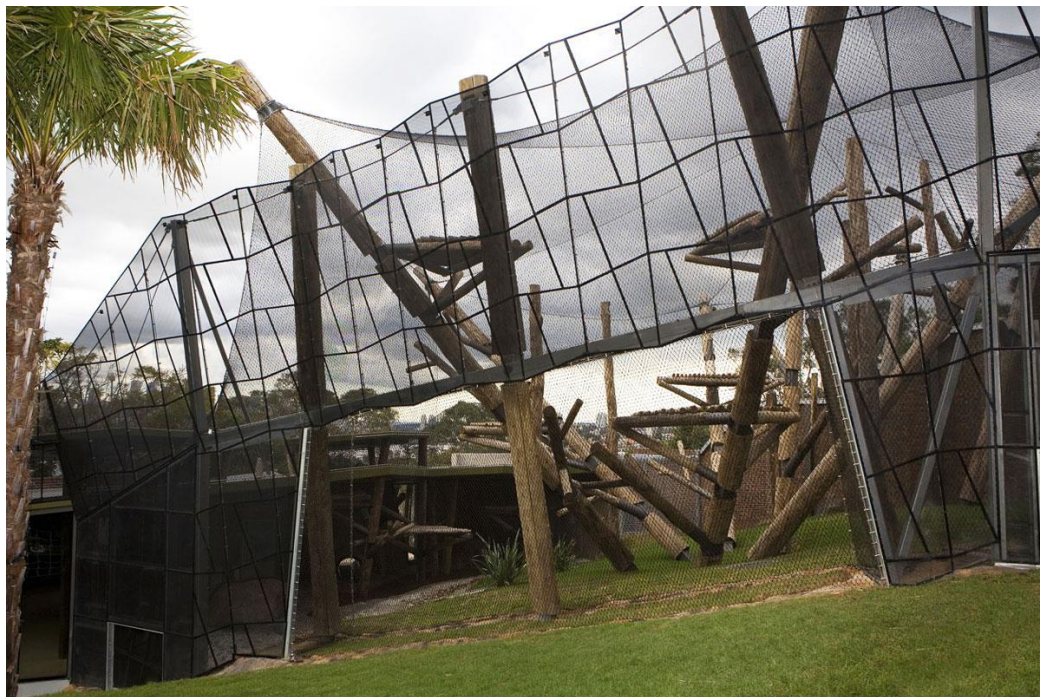
Fig. 1.1. Enclosure structure in Taronga Zoo, Sydney (Australia). (Image by Ronstan Tensile Architecture)
