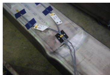
Fig. 4.36. Detailed view of the local failure of specimen S4 – EC1.
