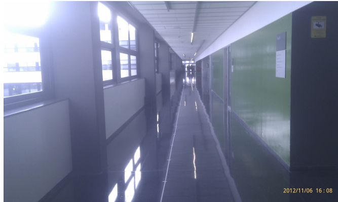
Figure 3.11: Indoor propagation environment. The outer of the building and the floor partitions are made by reinforced concrete, whereas the wall partitions are made by plaster and the floor is made of stoneware. Finally, it is important to mention that there are metal structure in the ceilings used to conduct the electricity and communications wiring.
