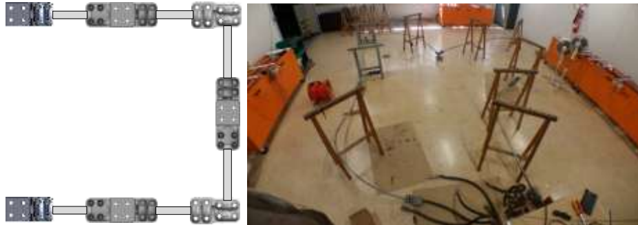
Figure 6.4. Experimental setup of the proposed temperature rise test performed to validate high-capacity substation connectors. The terminals placed at both the extremities of testing loop are making the connection with the power transformer and are not object of the test.
