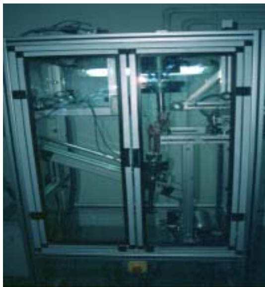
Figure 15: Picture Of The Simulator Control System Composed By A Control Station.
