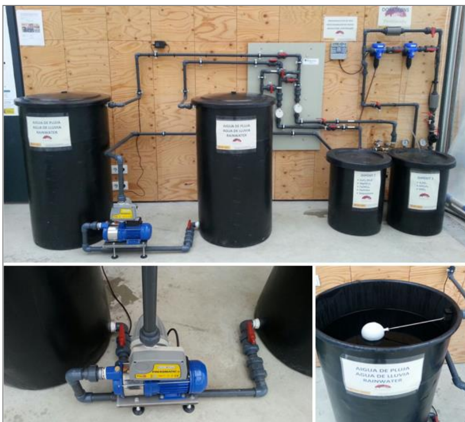
Figure 2.14 Final irrigation system of the i-RTG (top), water pump of the greenhouse (bottom left) and interior of a water tank with a buoy mechanism (bottom right).
