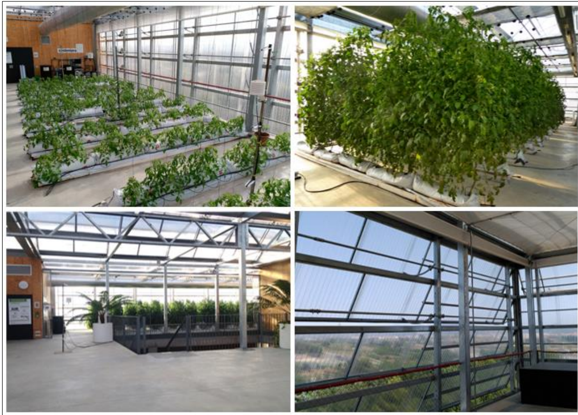
Figure 8.2 i-RTG with a crop of two weeks (top left), i-RTG with a crop of four months (top right), i-RTG from the atrium (bottom left), and polycarbonate sheets in the wall of the greenhouse (bottom right).
