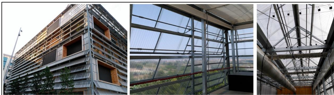
Figure 7.2 ICTA-ICP building in the UAB Campus (left), walls of the greenhouse (centre), roof of the greenhouse (right).
