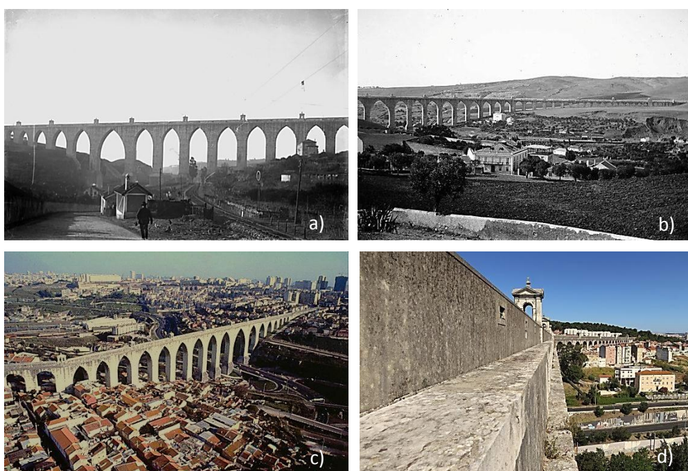
Fig. 35 – Lisbon Aqueduct in Alcântara valley: a) in 1912 (source - Arquivo Municipal de Lisboa: doc. PT/AMLSB/PAG/000402); b) in 1930 (source - Arquivo Municipal de Lisboa: doc. PT/AMLSB/PAG/000401); c) in 2013 (source - FCT-UNL at URL http://eventos.fct.unl.pt/enterface13 ); d) in 2015 (source - from author).
