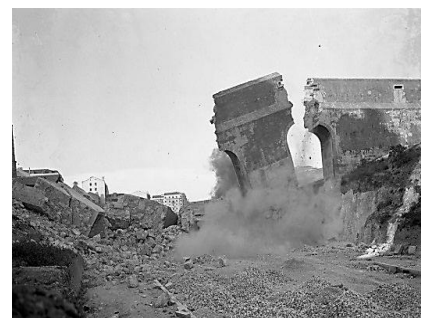
Fig. 40 – Aqueduct demolition to give space to what would be nowadays Infante Santo Street. 1949. (source - AML: PT_AMLSB_FMC_000006).
