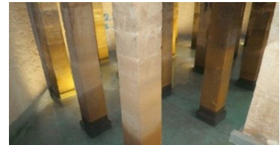
Fig. 38 – Patriarcal reservoir (interior).
