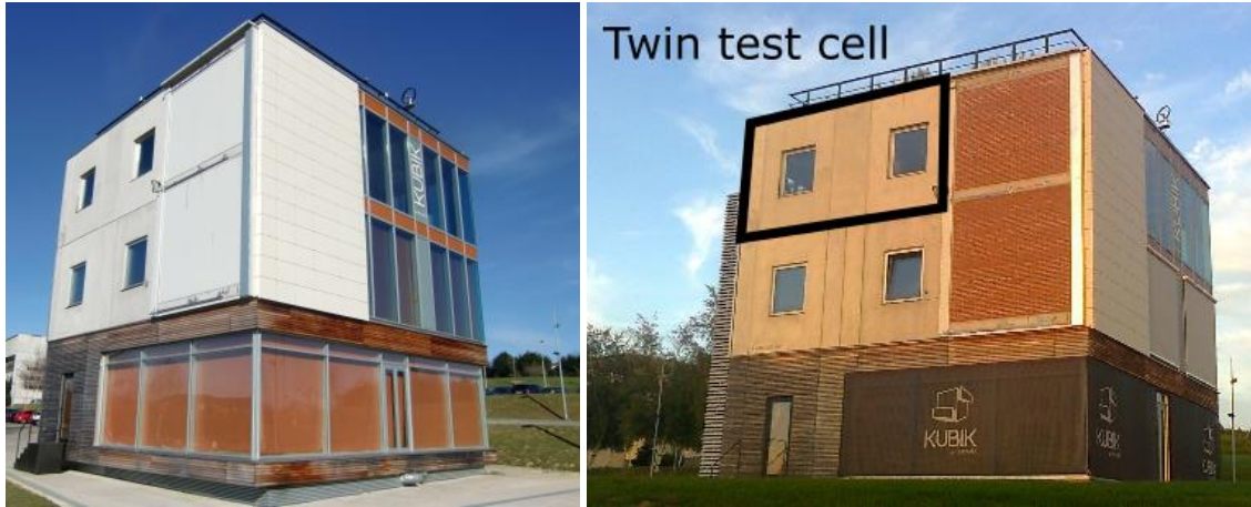
Figure 5: South-West view of the KUBIK test facility (left) and location of the test cell for testing of indoor insulation systems (right).
