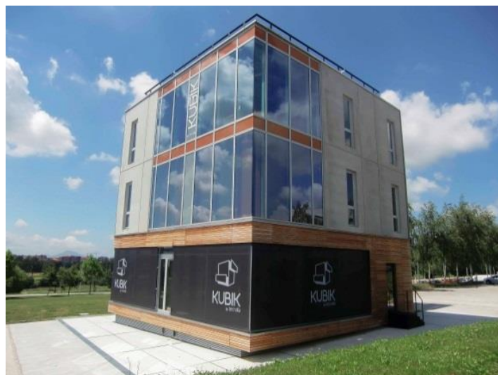
Figure 1: External view of the Kubik by Tecnia test facility
