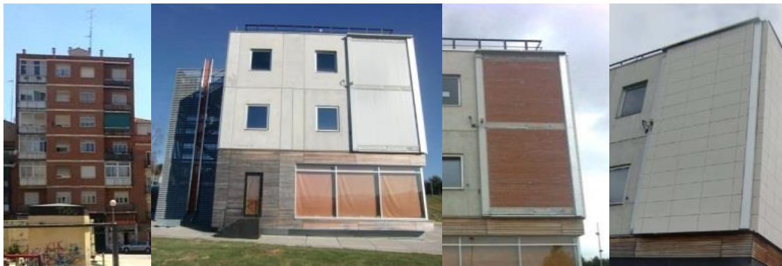
Figure 3. Left: Building with brick façade, Center-left: Calibration façade test configuration in KUBIK (phase 0), Center-right: Brick façade test configuration in KUBIK (phase 1), Right: Ventiladed façade solution in KUBIK (phase 2)
