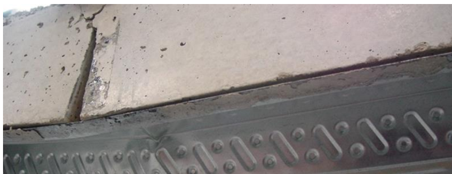
Figure 5.38 Vertical disconnection observed at the laboratory specimen
