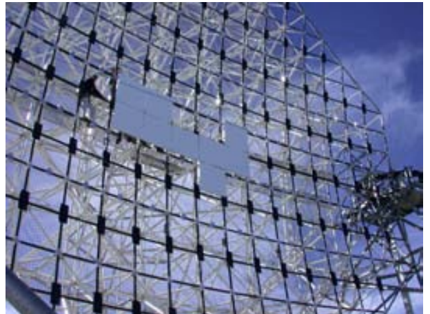
Figure 2.8: MAGIC space frame structure.
