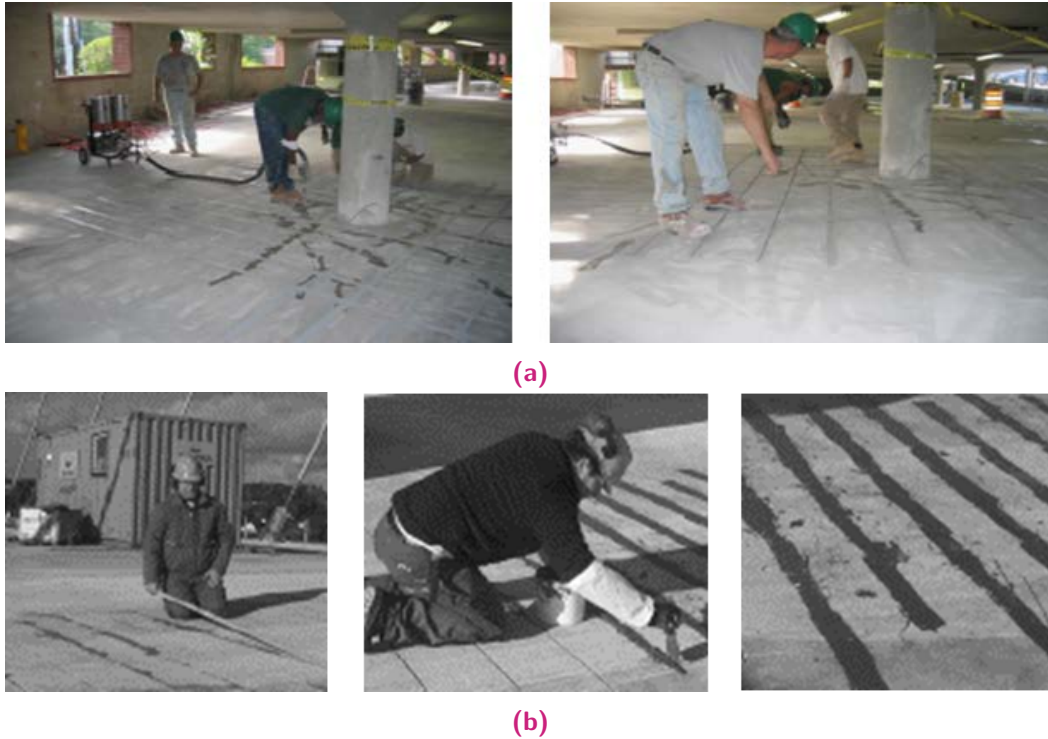
Figure 2.10: NSM applications (a) Strengthening of parking garage decks [46] and (b) Strengthening of bridge in Sweden [23].
