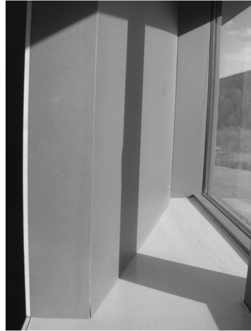
Figure 7. Absorption panel on the south-oriented façade.
