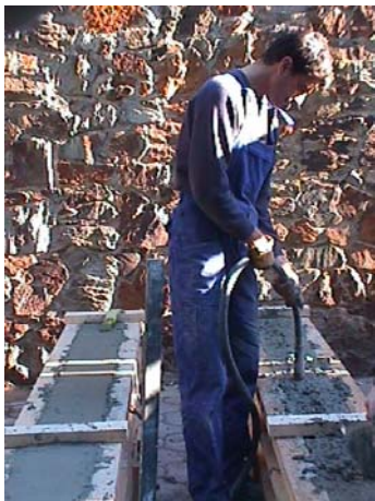
Compacting the fresh concrete
