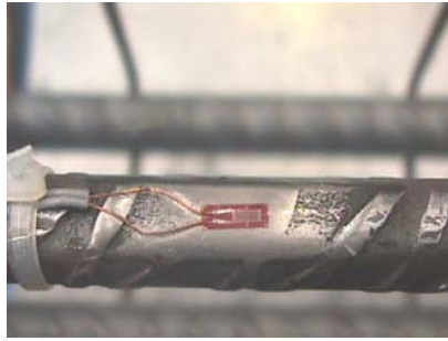
Fig.5.7: Strain gauges in the reinforcement
