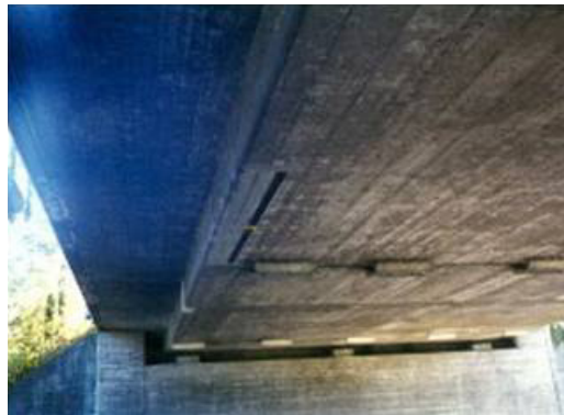
Figure 1.1. Strengthening of the Ibach Bridge in 1991 in Switzerland. (Cress, 2000)
