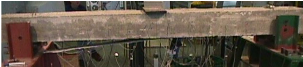
Figure C.24. Peeling failure in Beam 1/B initiated around flexural or shear cracks.
