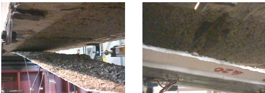
Figure C.31. Possible crack location of the debonding initiation. Visible stirrup after failure in Beam 1/A.
