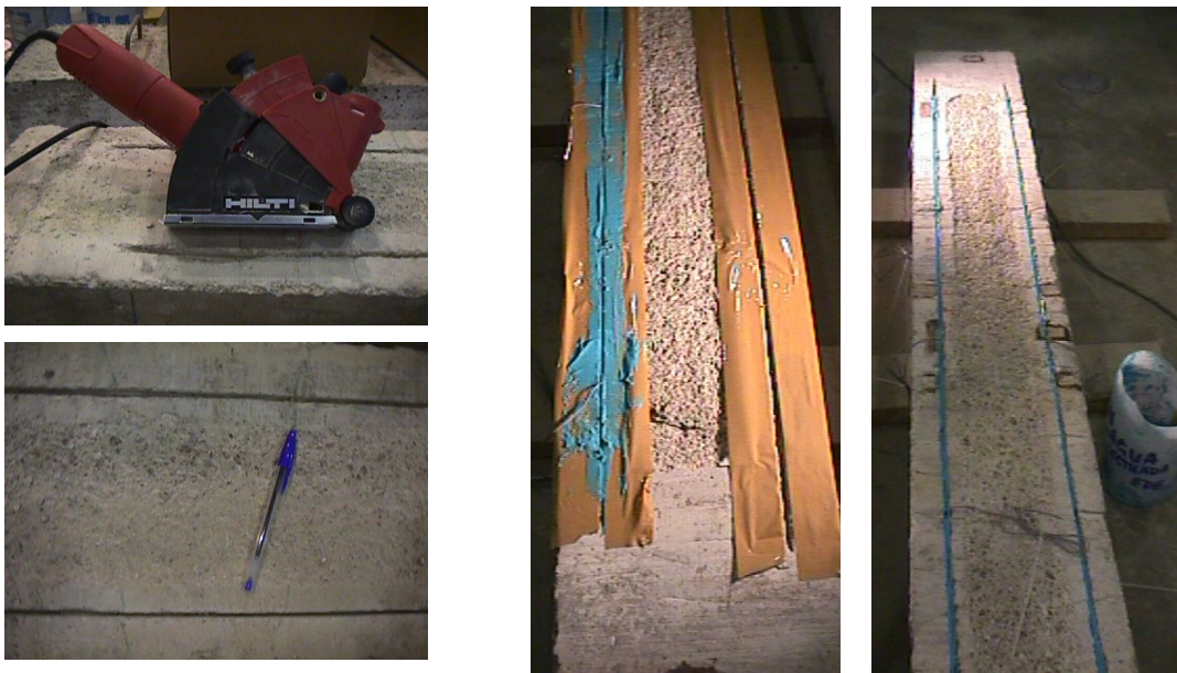
Figure C.85. Two slot-applied laminates were bonded in Beam 1/B (#2).
