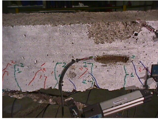
Figure C.48. Concrete crushed near the load application point for a load level close to failure.
