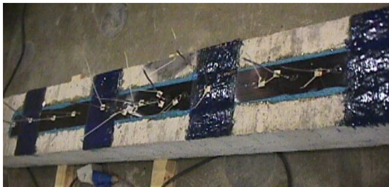
Figure C.61. External anchorages applied only on the bottom side of Beam 2/A.
