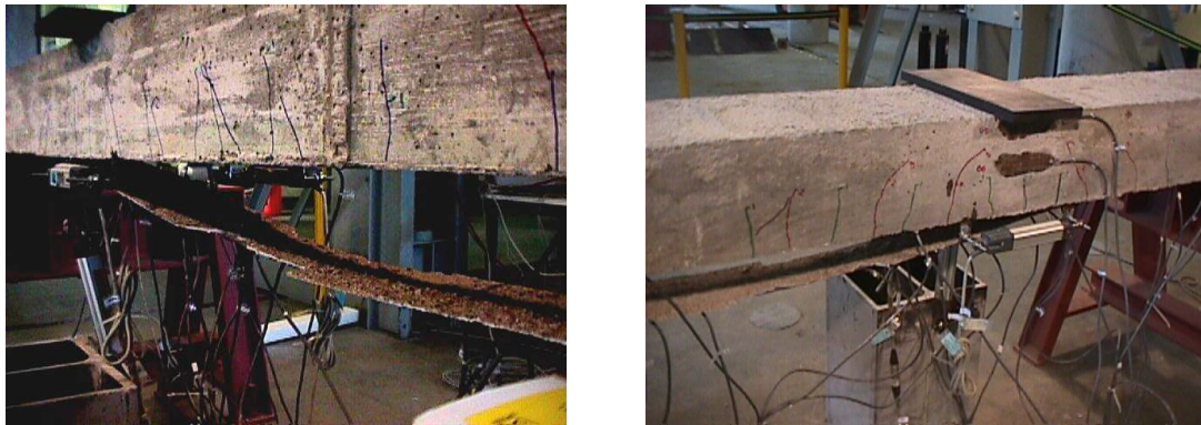
Figure C.30. Peeling failure in Beam 1/A initiated near midspan.
