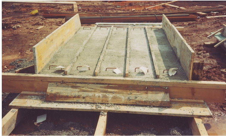
Figure C.2. Casting of the beam specimens.
