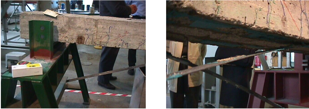
Figure C.68. Laminate 1 peeled-off without the detachment of a concrete cover layer in more than half of the debonded laminate.
