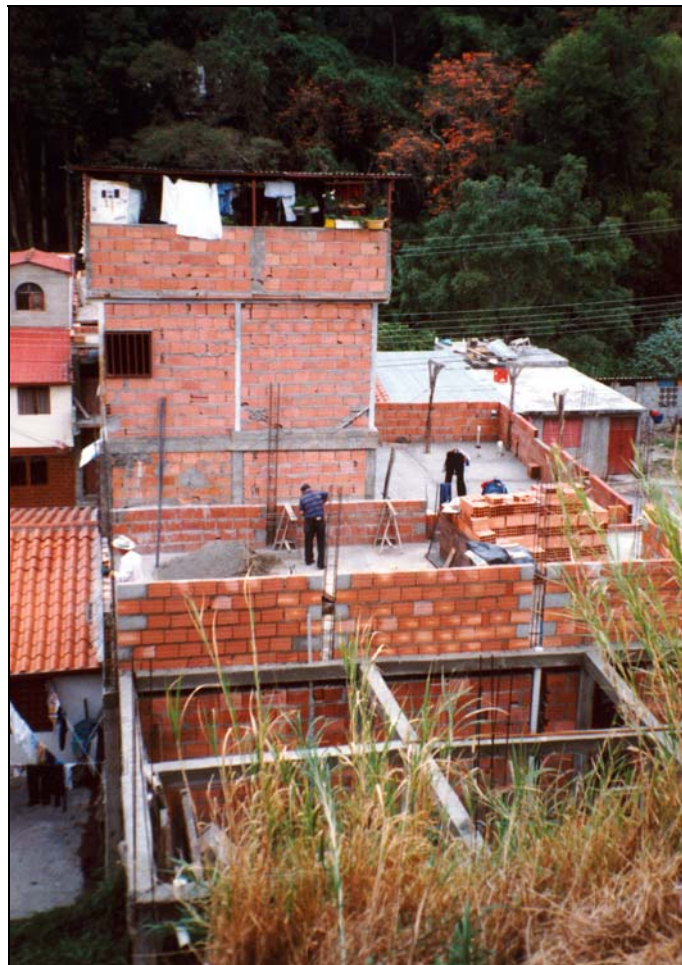
Picture 18: Building under construction
