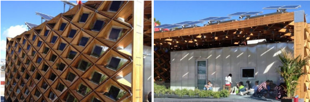
Fig. 3. 1 The Eco-House prototype exhibited at SDE 2012. BIPV systems are used in the façade and BAPV on the roof.
