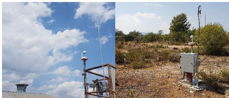
Fig. 4. Sharp grounded rod installed in the two setups: rooftop (left) and flat-ground (right).
