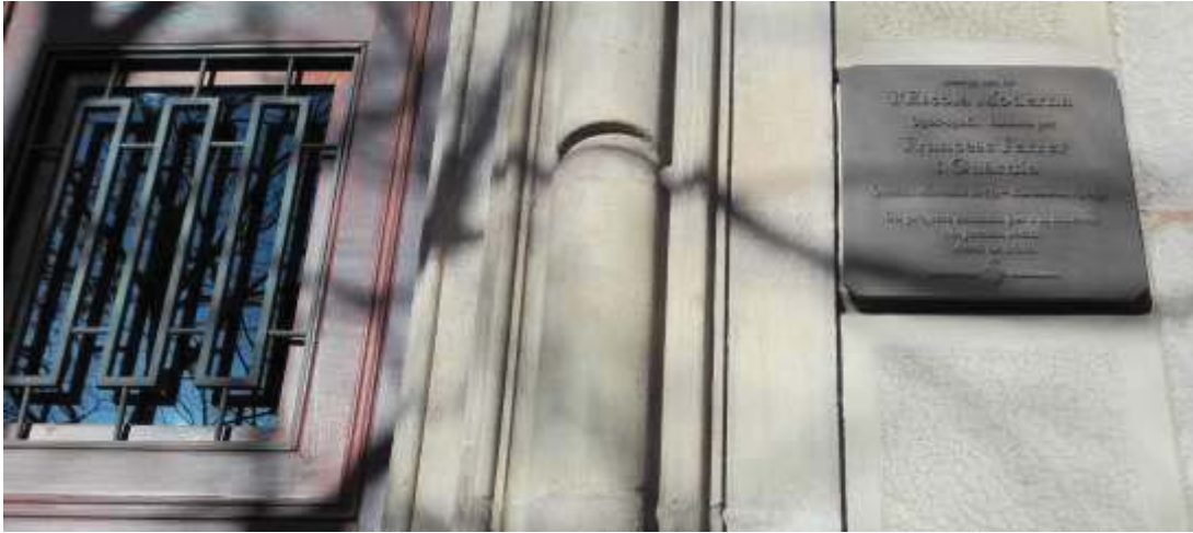
Figure 2: Front Door of the Modern School, Bailèn street, Barcelona
