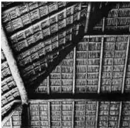
Katsura Villa, Kyoto, End of 16th to mind 17th century. Bamboo roof construction over open space. (Nitschke 1988, p. 37.)
