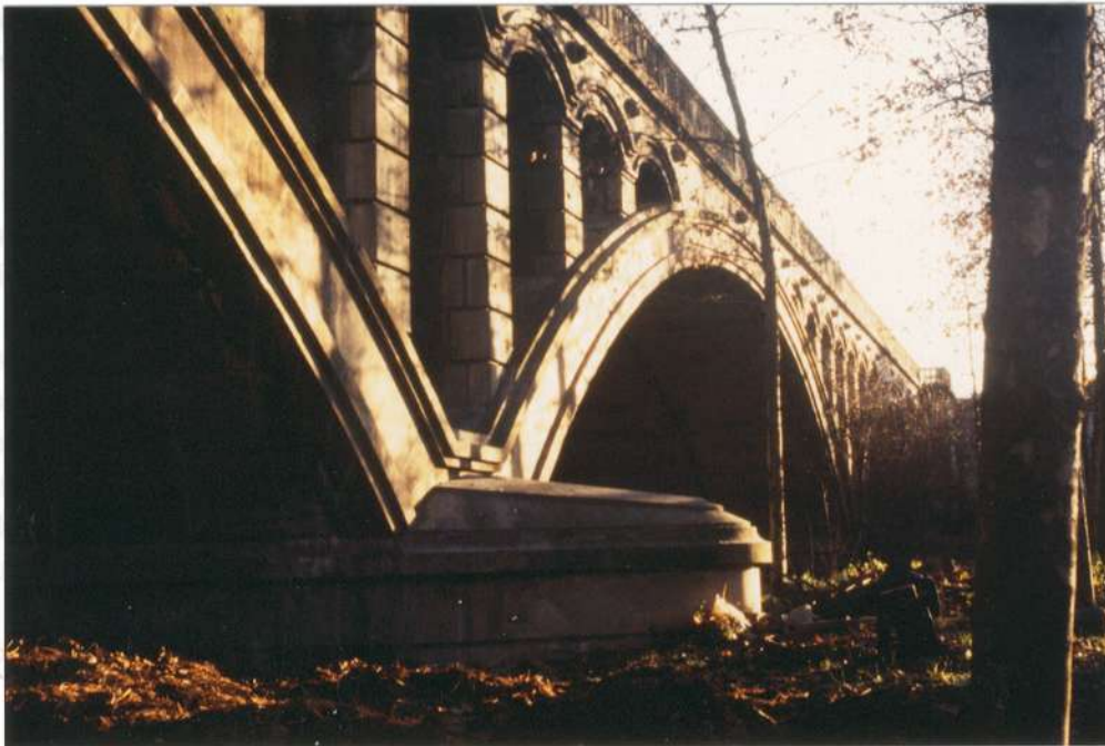
Exterior view of the historic stone bridge, showing the multiple arches and the surrounding landscape with trees and foliage.
