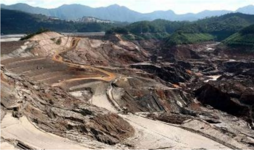
Figure 2.17 The 110-meter high Fundão mine tailings dam in Minas Gerais collapsed. Image Credits: ©Fonseca do Carmo, 2017.
