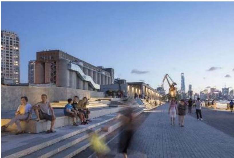
Figure 6.4 Renovation of 80,000 tons of silo at Shanghai Minsheng Pier
