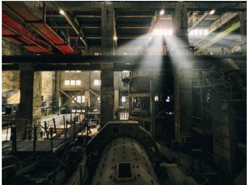
Figure 4.6 Interior space of Huaxin Cement Plant
