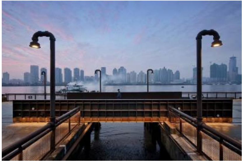
Figure 6.6 Water pipe light Image Credits: ©Ronghua Luo, 2020.
