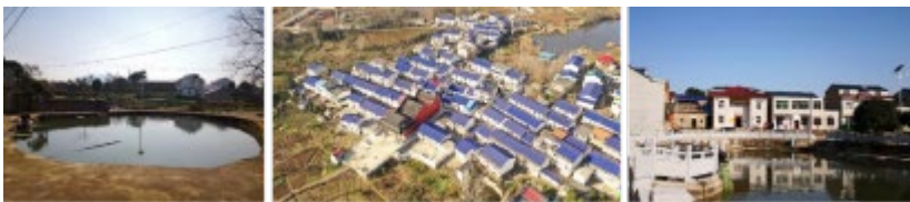
Figure 5.23 Traditional village architecture and its layout Left: village pond. Middle: village layout. Right: ancestral hall. Image Credits: ©Qipeng Liao, 2021.
