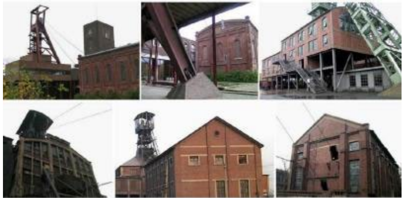
Figure 2.8 Characteristic coal mine wellhead house and winch house.
