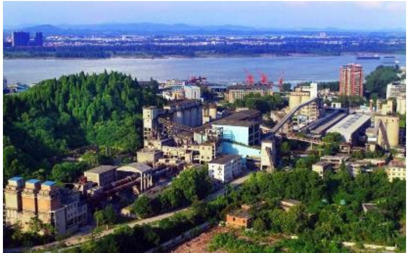
Figure 4.1 The Huaxin Cement Plant.
